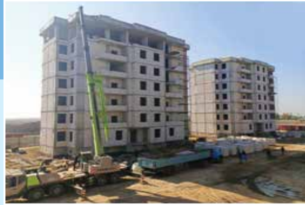
Image 3: Use of AAC in High Rise Building
